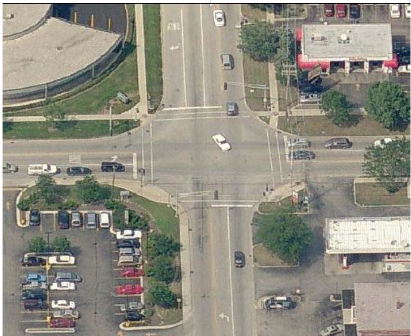
The Greenwood Rd. and Glenview Rd. Intersection in the Village of Glenview is programmed for an intersection improvement in FFY 10. The project is scheduled for a March 2010 letting
