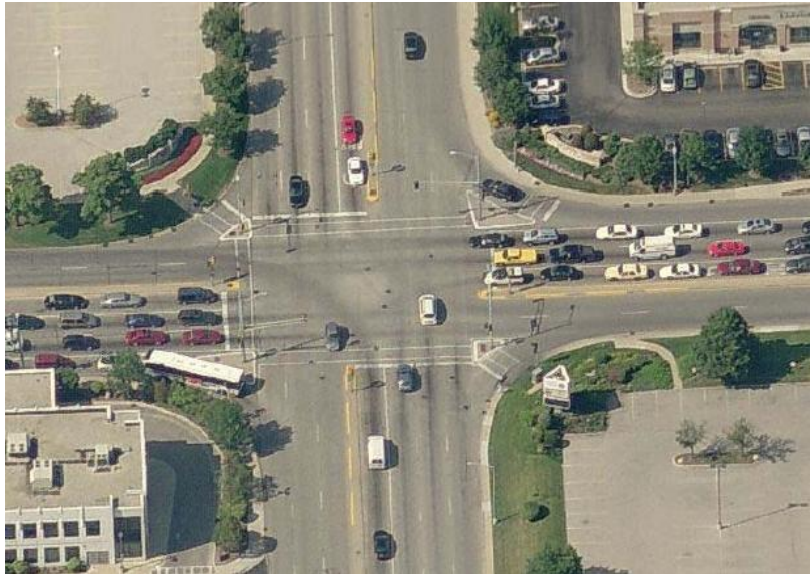
The Golf Rd. and Skokie Blvd. Intersection in the Village of Skokie is programmed for an intersection improvement in FFY 2010. The project is on the November letting.
