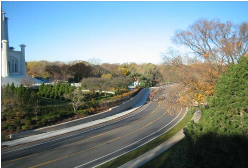
Completed Segment of Sheridan Road—courtesy of Wilmette
